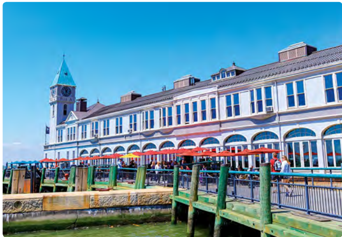
Pier A Harbor House
